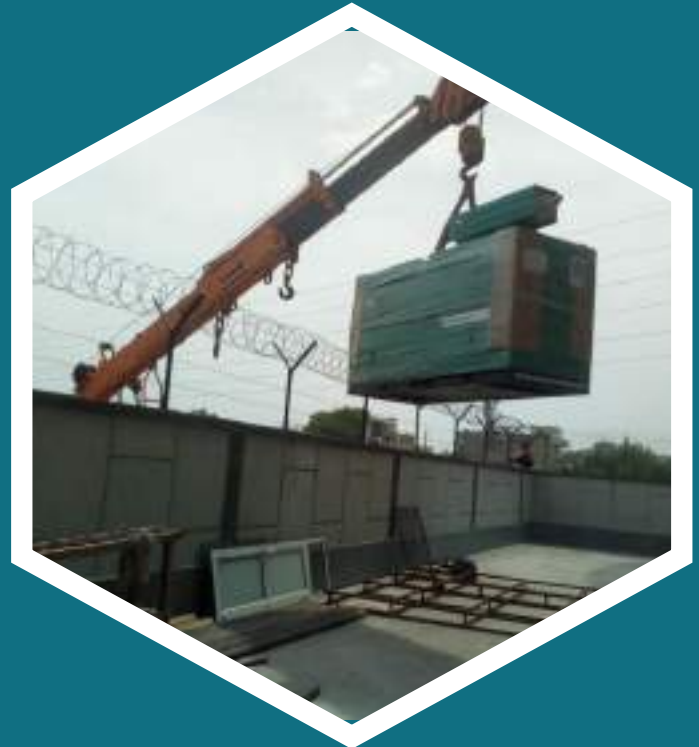
A 62.5 KVA DG set lifted over the wall
