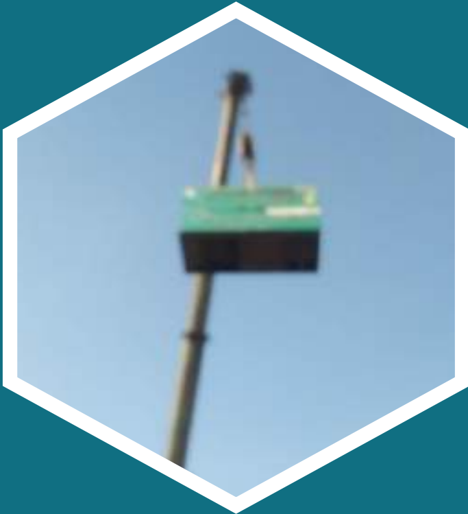
A 40 KVA DG set lifted on the rooftop
